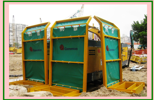
Equipment wrapped with noise barriers to minimise noise impact
