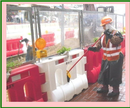
Regular washing at works area
